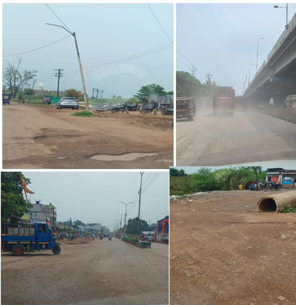
Figure 5.4: Broken roads causing higher road dust emissions.
