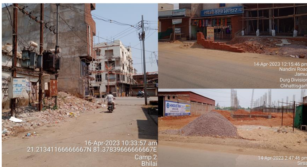
Figure 5.2: Construction material and debris near construction sites
